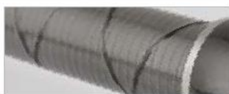
Carbon yarn reinforcement wrapping.
